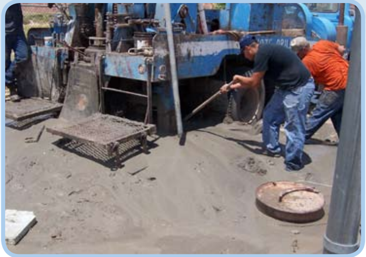
Workmen pump silt out of the well at La Vida Mission.
