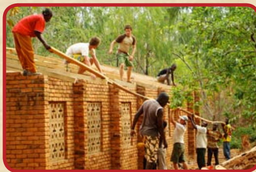
Bjorn's team lifts a roofing truss.
